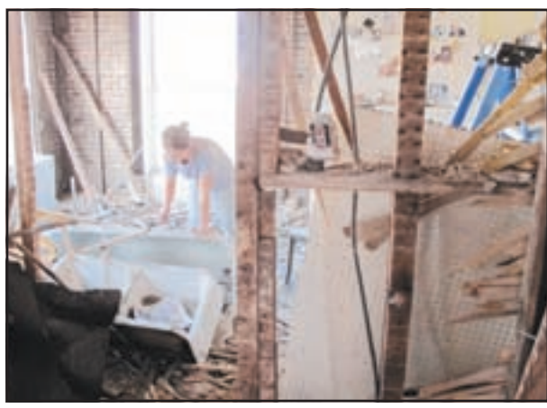
PICKING UP THE PIECES: Jadwiga Bronte says her landlord trashed her apartment on Bedford Avenue in an attempt to force her out. Photo by Ben Lockhart
