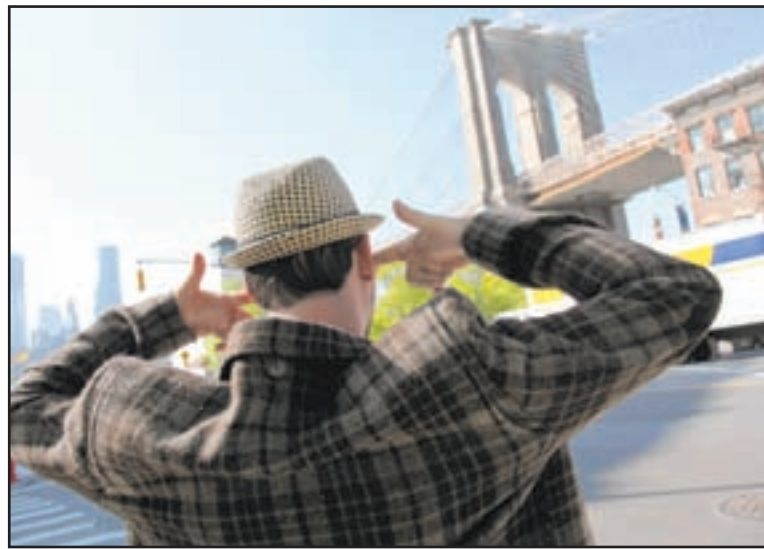
SOUND AND FURY: Neighbors of the Brooklyn Bridge say noisy drilling at the base of the span is keeping them awake all night. Photo by Bess Adler
