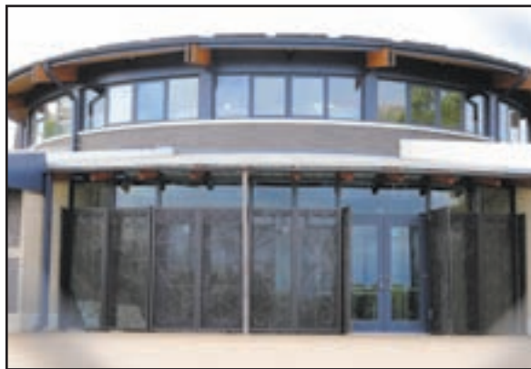
LEFT FALLOW: The Marine Park park house hadn't been worked on in more than six months, city officials say.
