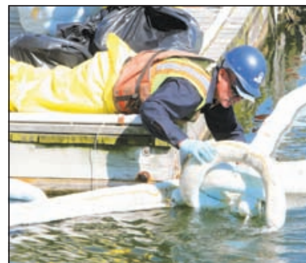
OIL WALL: City workers place a barrier, called a hard boom, in Paerdegat Basin following the Sept. 27 spill — a spill that some say was caused by firefighters who did not know what they were hoses off of Paerdegat Avenue North. Photo by Steve Solomonson
