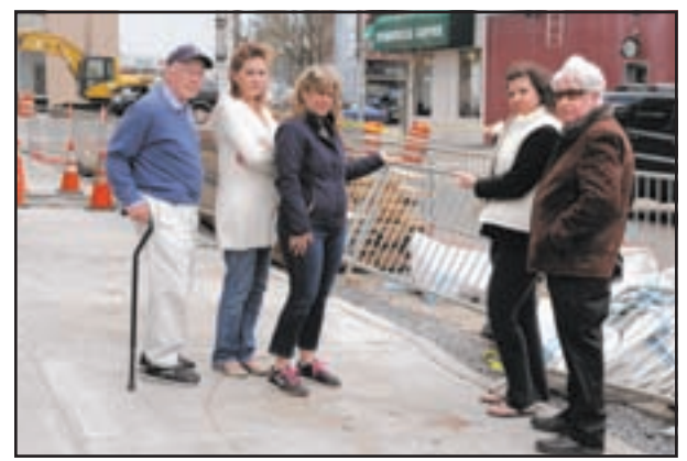
STILL IN THE HOLE: Neighbors along 92nd Street between Third Avenue and Ridge Boulevard say the repairs on their block are still ongoing 10 months after a massive sinkhole opened on the corner last summer. Photo by Bess Adler
