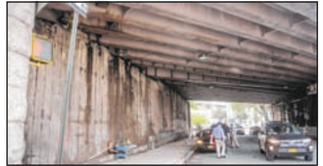
CRUMBLING: Department of Transportation officials have inspected the section of the bridge, and say it is safe. Photo by Stefano Giovannini
