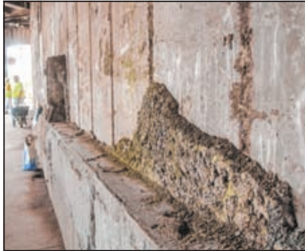
WALL FALL: The granite facade covering this section of wall underneath the Brooklyn Bridge collapsed onto the sidewalk the night of July 2, injuring three kids and two adults who were reportedly taking shelter under the bridge and waiting for last Wednesday's torrential downpour to subside. Photo by Stefano Giovannini
