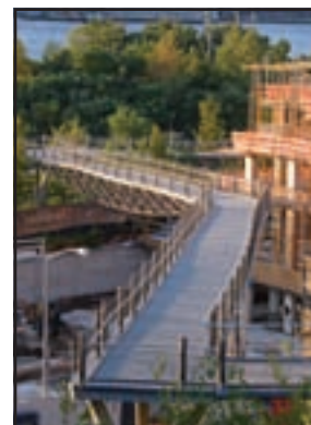
BOUNCED OUT: The hiking trail-like Squibb Bridge was made to bounce a bit as people passed over it, but it closed because it was bouncing too much.
