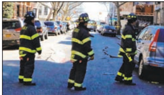
ALL THE CITY'S MEN: The sinkhole prompted a response from the fire and police departments, the Department of Environmental Protection, Con Edison, and National Grid. Photo by Steven Schnibbe
