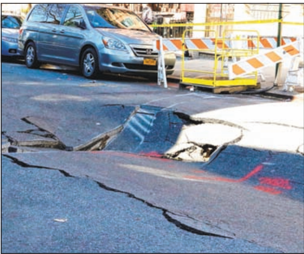
IT'S GETTING DEPRESSING: A sinkhole the length of three cars and half as wide as the street opened on 56th Street on March 1, prompting the city to shut down the block. Sunset Parkers now have to contend with two sinkholes just seven blocks away from each other. Photo by Steven Schnibbe
