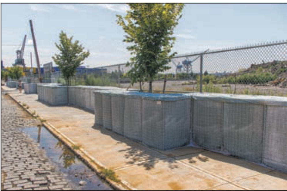
BUILDING WALLS: The city has finished installing this four-foot barrier along Beard Street, which is designed to protect Red Hook from minor flooding. Photo by Caleb Caldwell
