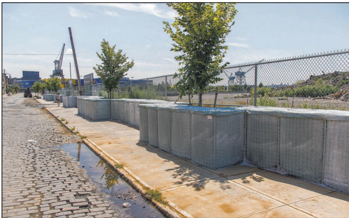
BUILDING WALLS: The city has finished installing this four-foot barrier along Beard Street, which is designed to protect Red Hook from minor flooding.
