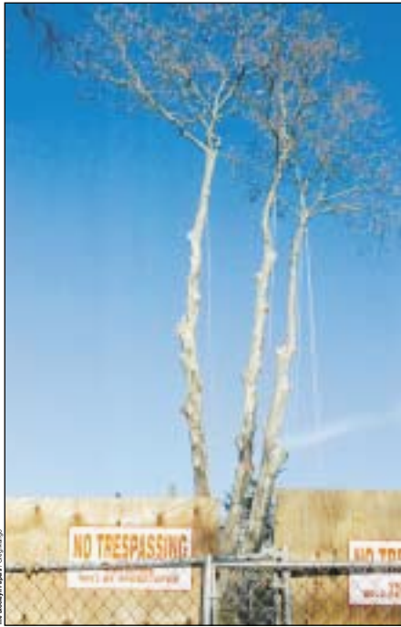
Not only has the home at 435 80th St. been demolished, but now this century-old tree, (what's left of it) was chopped down piece by piece this week.
