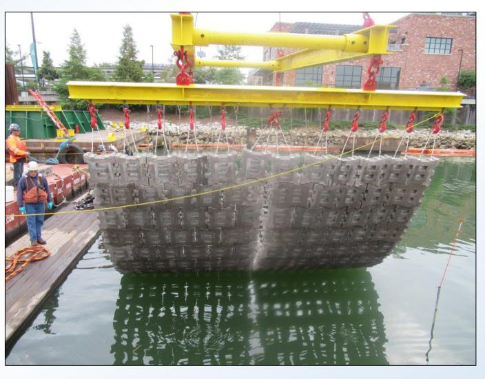
An armor layer consisting of open-celled articulated concrete blocks (ACBs) was installed on top of the sand isolation and filter layer to provide stability and protection of the cap. Underwater Divers made sure the ACB "mattresses" were placed and secured in the correct location.
