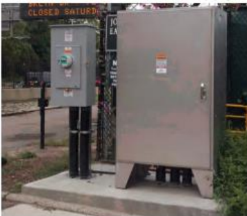
Proposed Electric Cabinet Enclosure for service (84"H. x 48"W. x 24" D.)
