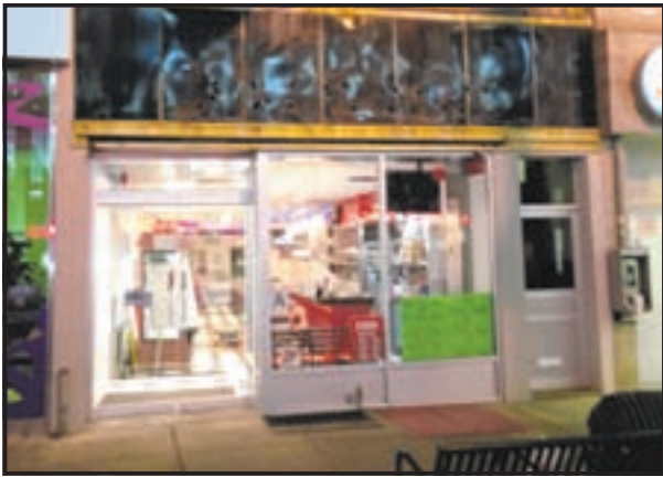
SIGN OF THE TIMES: New Hinsch's owner, Mike Moudatsos, said the classic sign over the entrance suffered damage during a cleaning of the exterior, and needed to be repaired. But he said Hinsch's old hanging sign was a public danger, and had to be replaced entirely. Community Newspaper Group \ Vince DiMiceli
