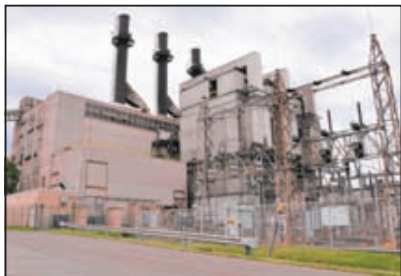
COMING DOWN: Goddard Power Plant, the last coal-fired power facility operated by the Navy, will be demolished and replaced by a natural gas plant.
