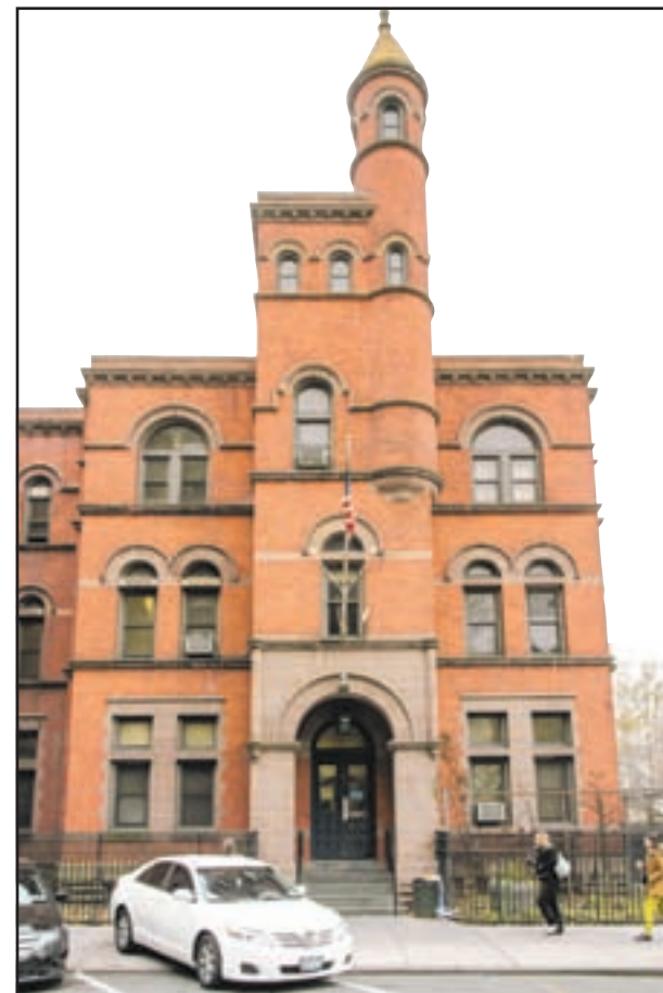
LANDMARK CASE: The 88th Precinct's station house on Classon Avenue in Clinton Hill will likely soon get landmark designation.
